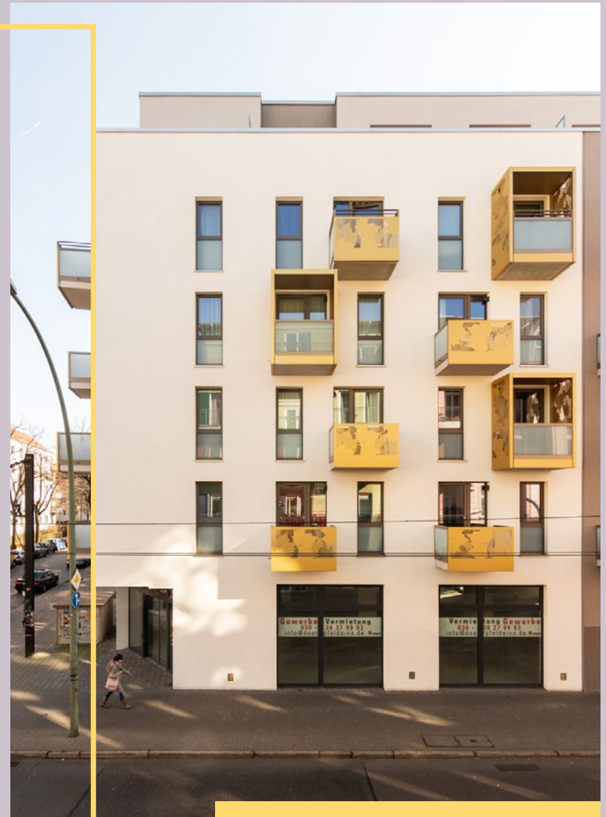
The front of the DP5 building has a stylish, assured appearance, with clear lines and sophisticated gold features.
